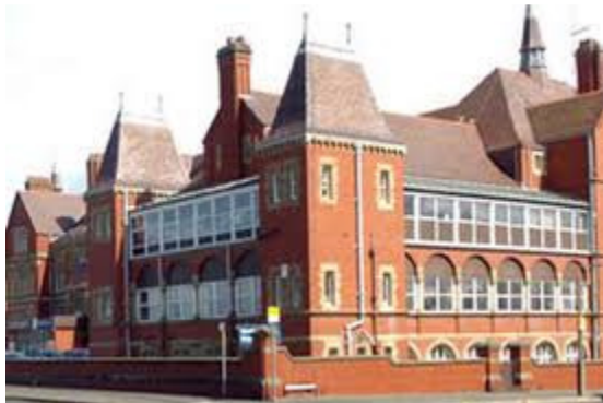
Site of North Denbighshire community hospital development
